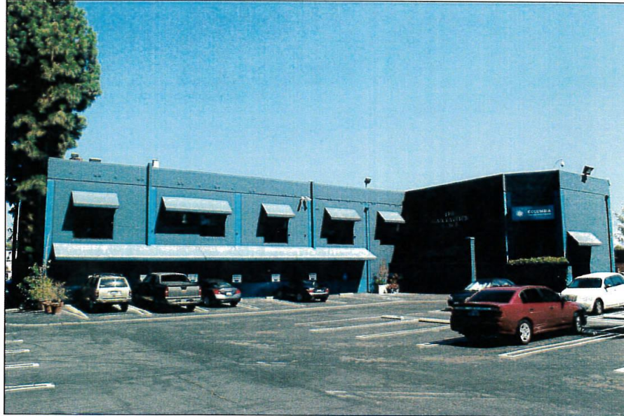
South elevation of subject, as viewed from parking lot
