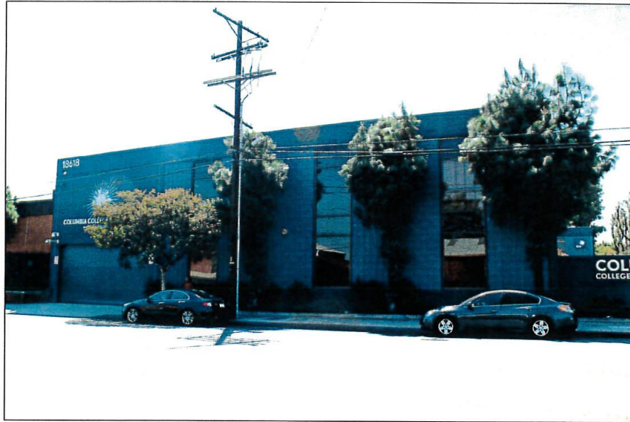
Front (north) elevation of subject, as seen looking south from Oxnard Street
