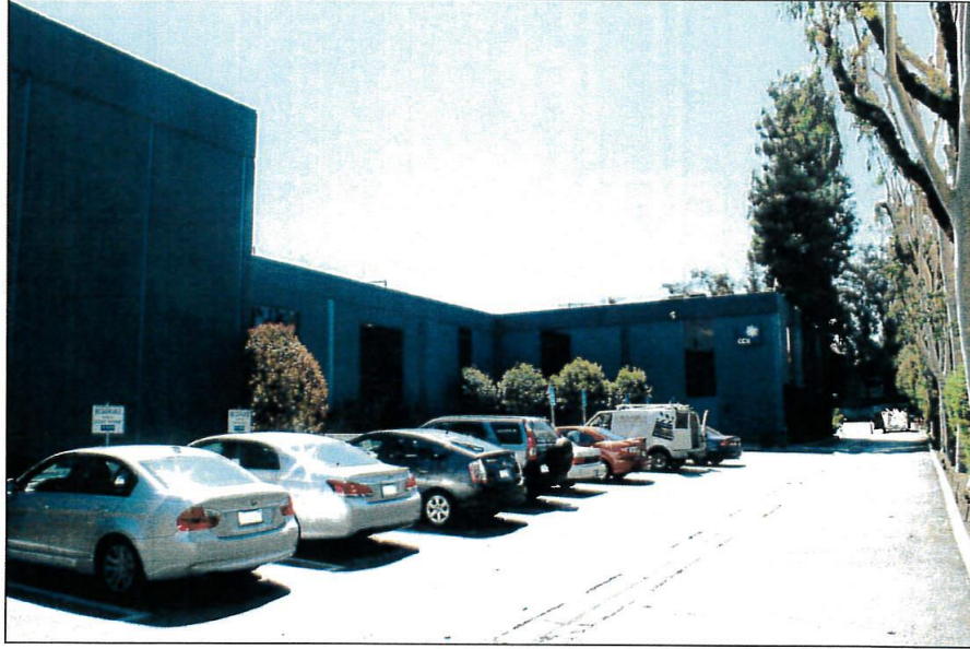
Subject's west elevation, as seen looking southeast from parking lot entrance
