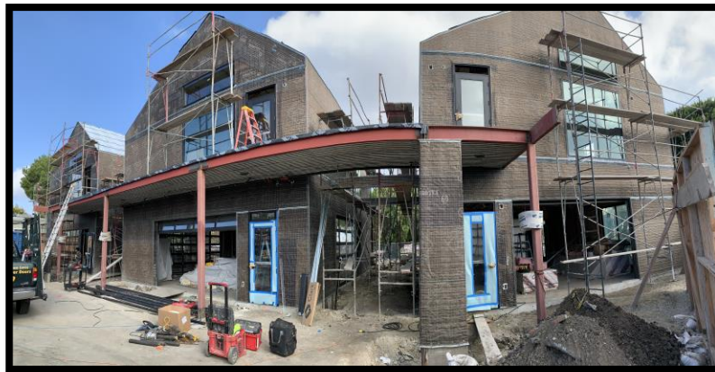
The Center for Innovation under construction
