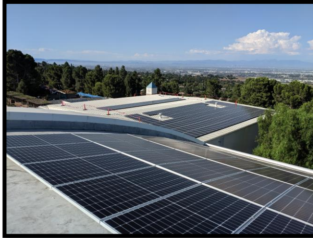
Solar Panels on the performing arts center
